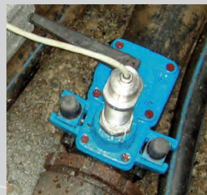
Installation via pipe saddle
