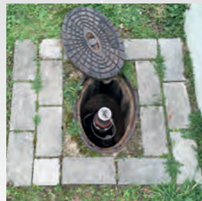
Installation via underfloor hydrant
